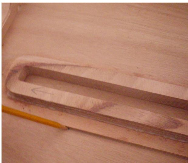
Mark the back edge of the opening, align the baseplate and spacer assembly on your mark, and trace the perimeter of the baseplate on the bottom panel.
